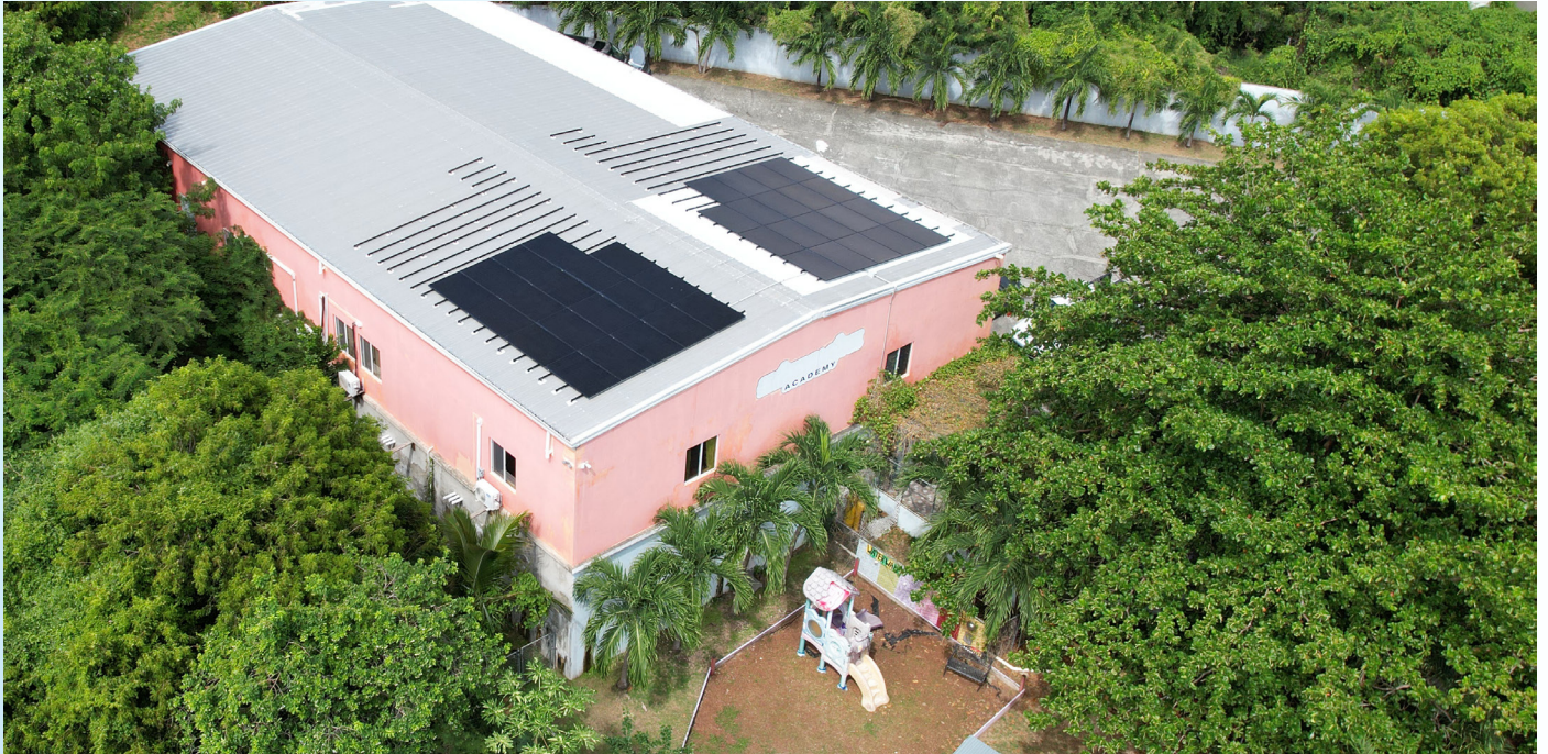
The Happy Faces II Academy will be the first of nine childcare centers that VIEO will harden with solar electric systems and battery energy storage solutions thanks to the Community Electrical Innovations grant program. (Photo by Eliji Mondesir).
