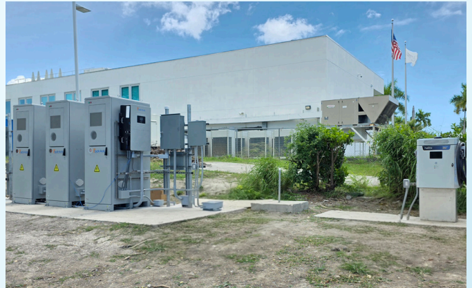
The first DC fast charger in the territory is located at the University of the Virgin Islands Research and Technology Park. (Photo by Kyle Fleming).
