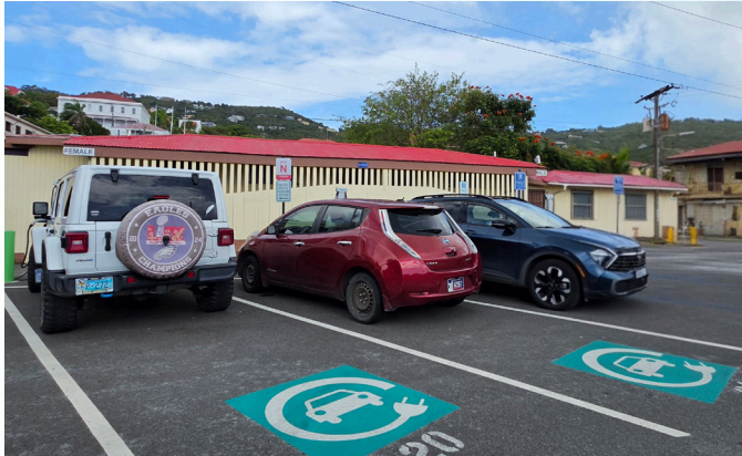
An EV charges up at one of six newly installed chargers located in the Fort Christian parking lot on St. Thomas. (Photo by Kyle Fleming).
