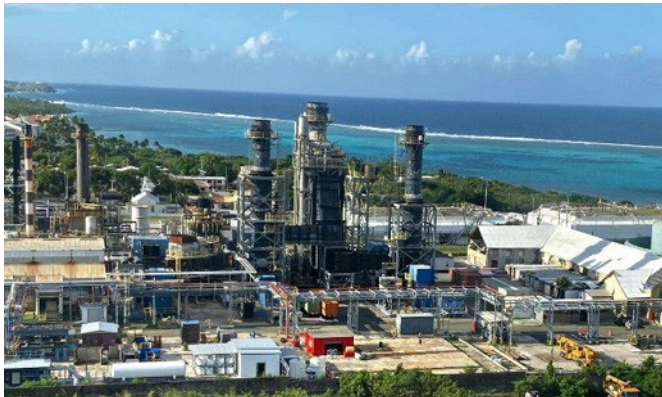
Figure 5. Estate Richmond Generating Station
