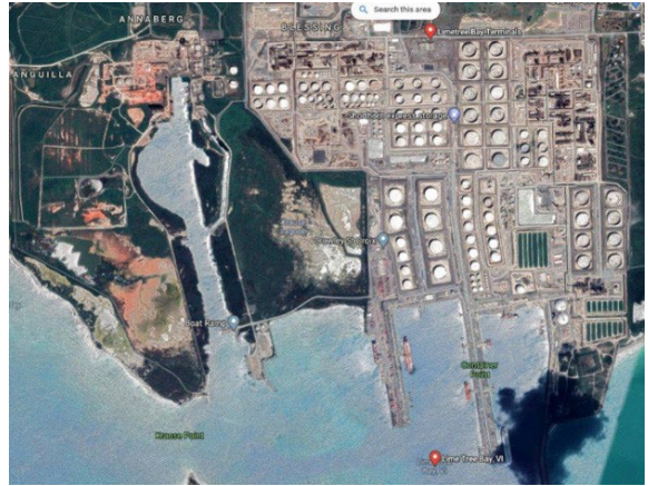
Figure 20. Limetree Bay Refinery and Terminal on St. Croix
