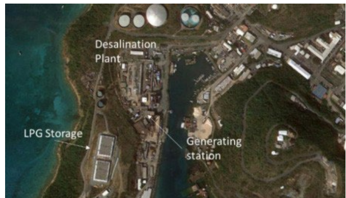
Figure 6. Randolph Harley Power Plant
